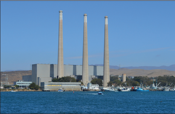
A desalination plant on the coast.
