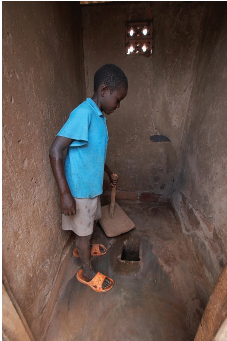
Figure 19 – A pit latrine. The waste falls into a pit.
